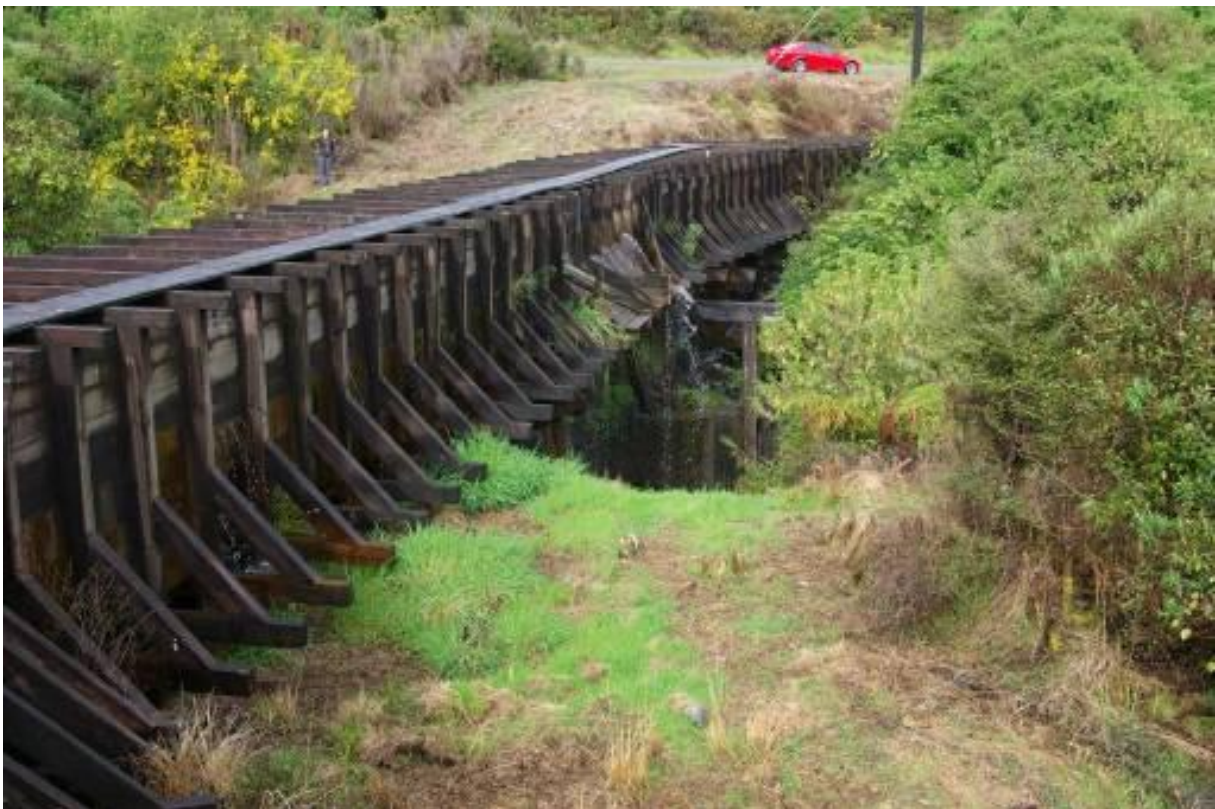
Figure 13. Fluming of the McKays water race over Coal Creek
