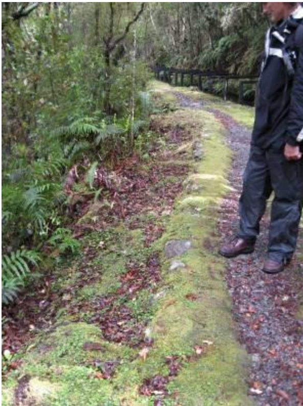
Figure 7. An example of successive repairs to the race with earlier posts holding timber retaining and subsequent timber boxing to hold that retaining
