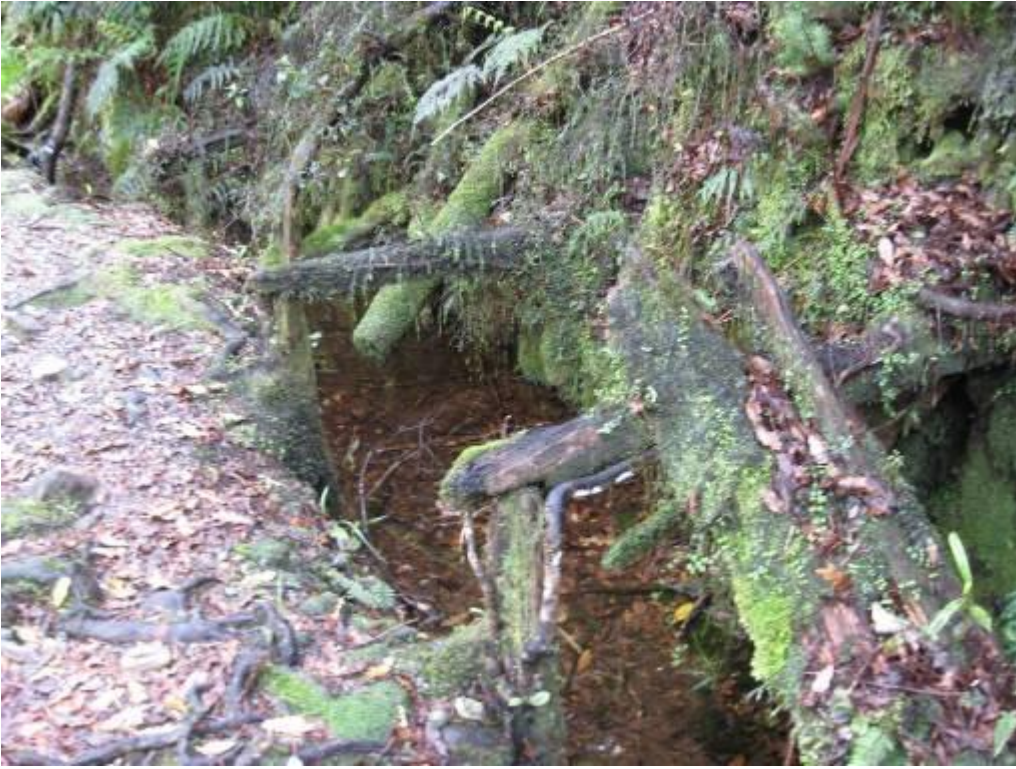
Figure 10. Original disused water race in the Wards Road to Kennedy Creek section, with old boxing timbers
