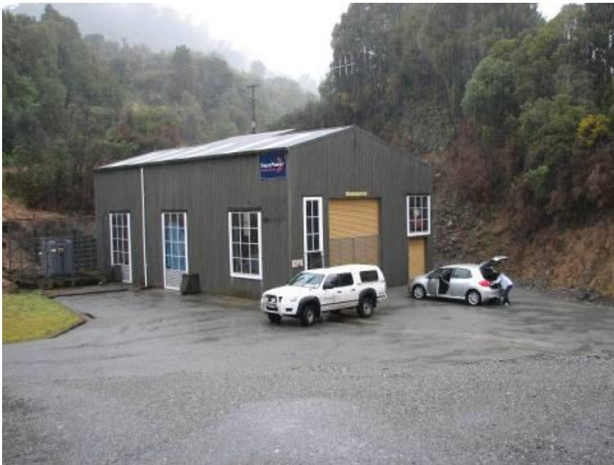
Figure 11. The original Kanierie Power Station and intake pipes (DOC West Coast Conservancy Photo Collection), and the rebuilt Kanierie Power Station today
