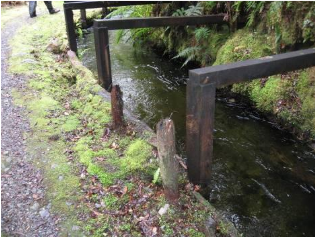
Figure 7. An example of successive repairs to the race with earlier posts holding timber retaining and subsequent timber boxing to hold that retaining
