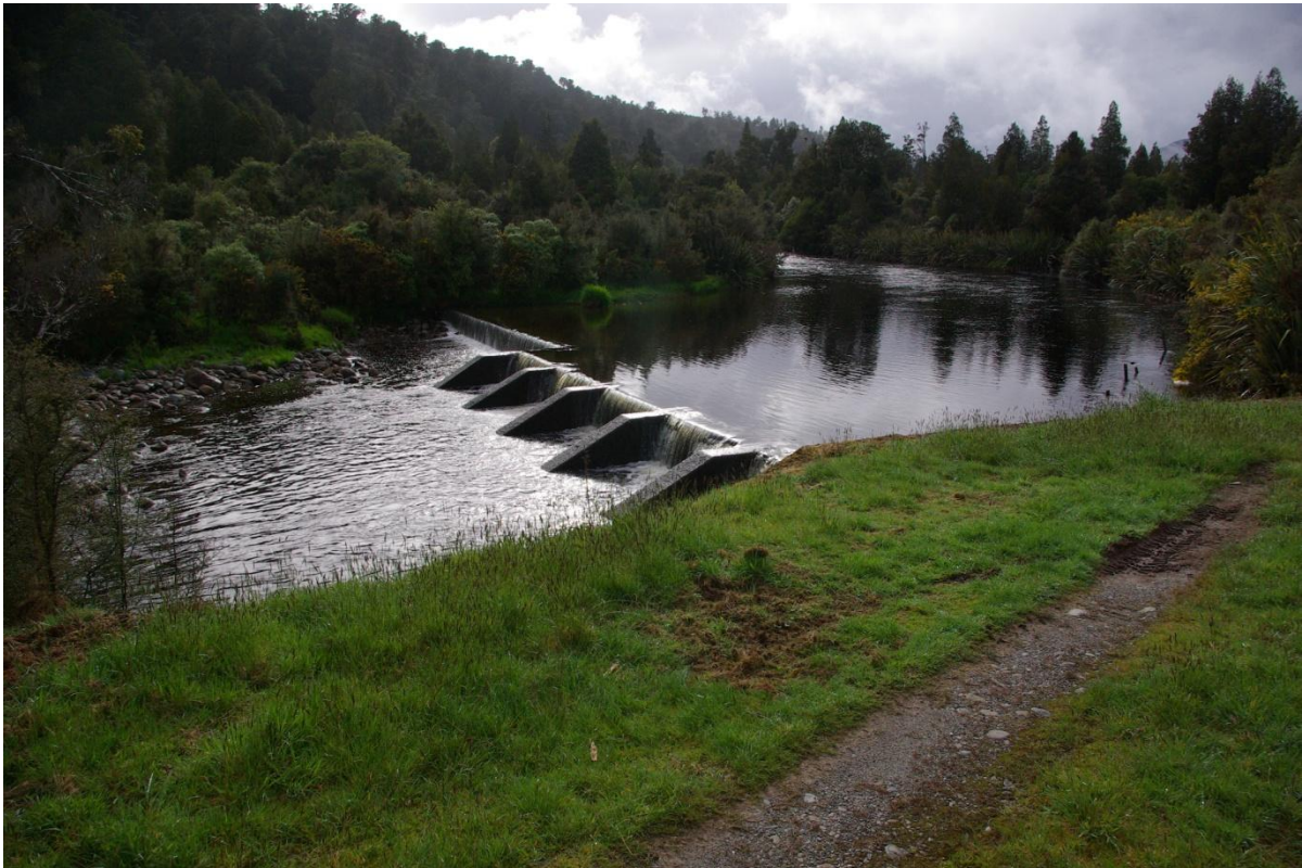
Figure 15. Weir at McKays
