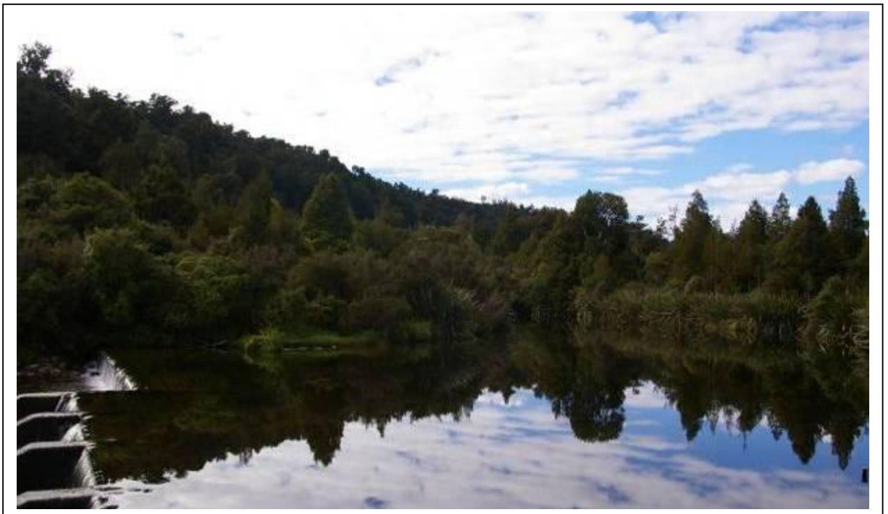
Photograph 13 – McKays impoundment Full flow (Photo 3279 10/11 April 2010)
