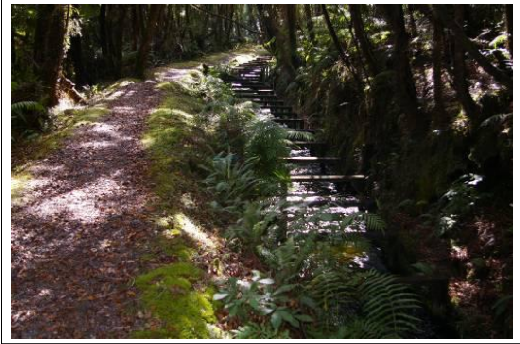
Photograph 6 – Kaniere Race adjacent to DoC walkway (Photo 3320 11 April 2010)
