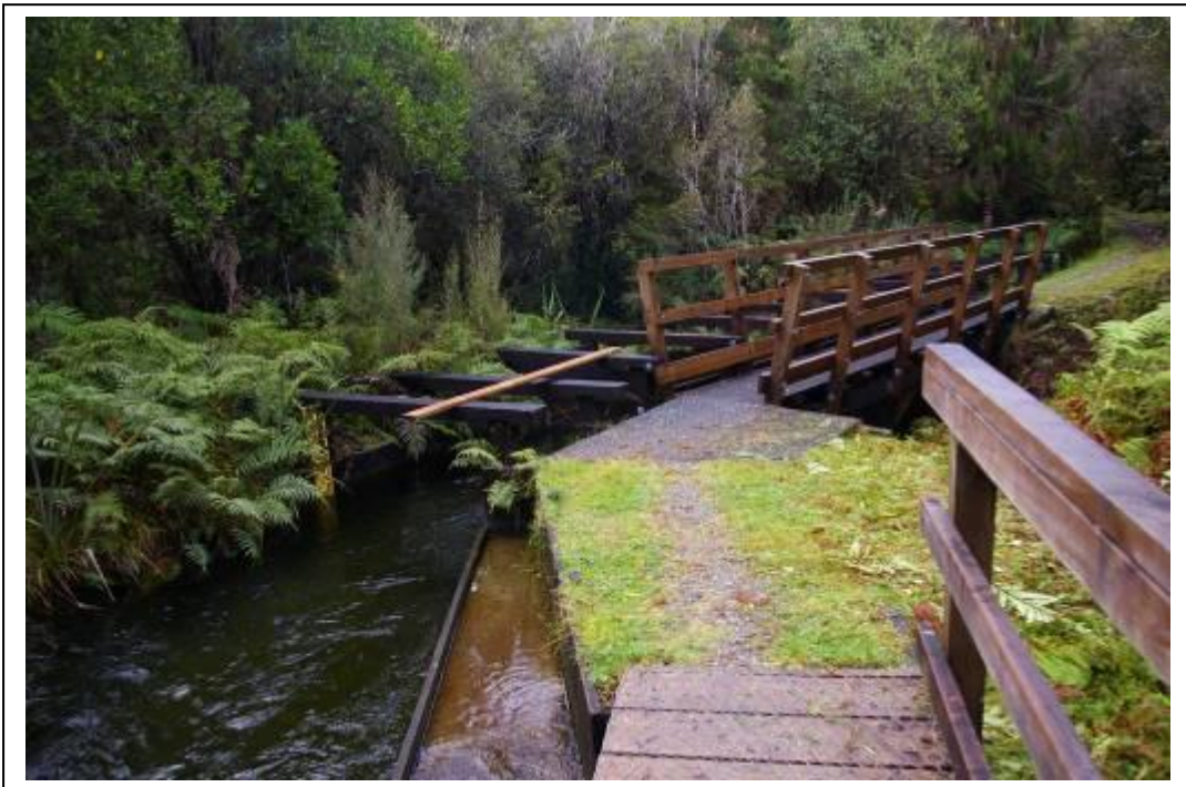
Photograph 7 – Kaniere Race, flume and bridges (Photo 3420 May 2010)
