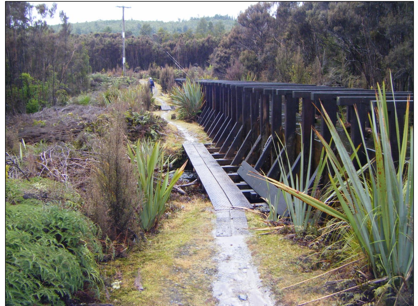
Photo of existing Kaniere water race and mountain bike route
