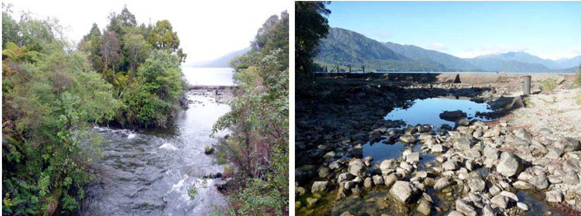
Figure 6.2 Left: Two channels at the Lake Kaniere outlet. Right: Control boards and concrete weir at Lake Kaniere outlet to true left channel.
