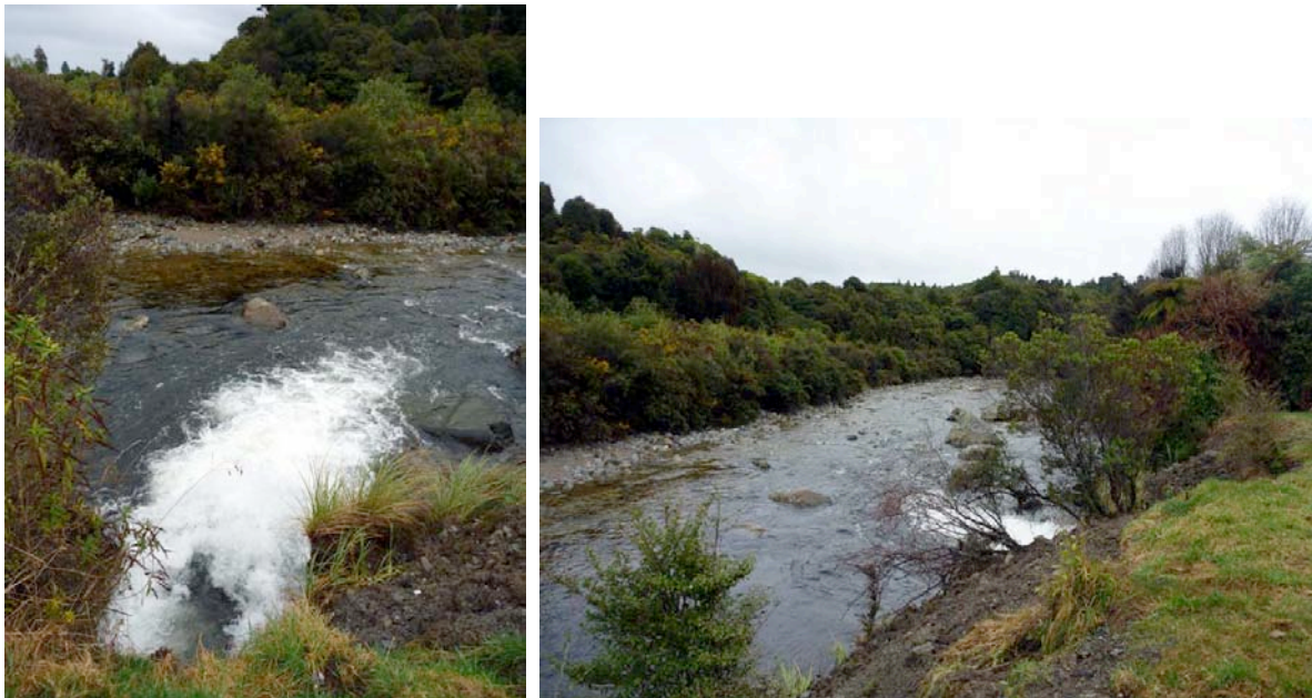
Figure 1.4 Kaniere Forks power station discharge to the Kaniere River.
