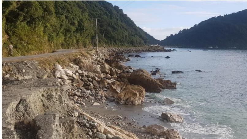
Figure 49: Coastal erosion and shoreline protection at Jackson Bay
