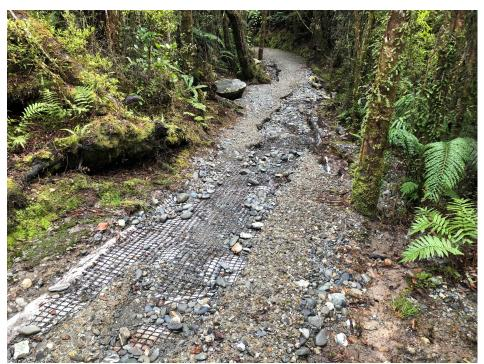
Figure 21: Trail Surface Damage
