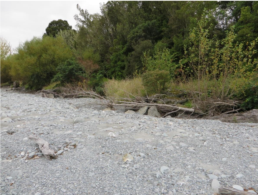
Figure 12: Partial submergence of snub groyne structures along right bank of Waiho River providing bank erosion protection upstream of Franz Josef Village WWTP
