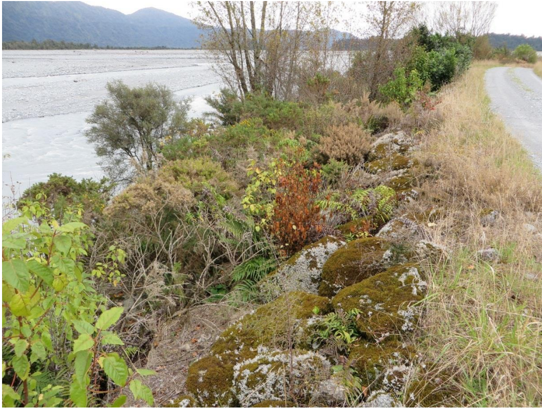
Figure 2: Rock armoured stopbank along right bank of Waiho River alluvial fan adjacent to oxidation ponds at Franz Josef Village WWTP
