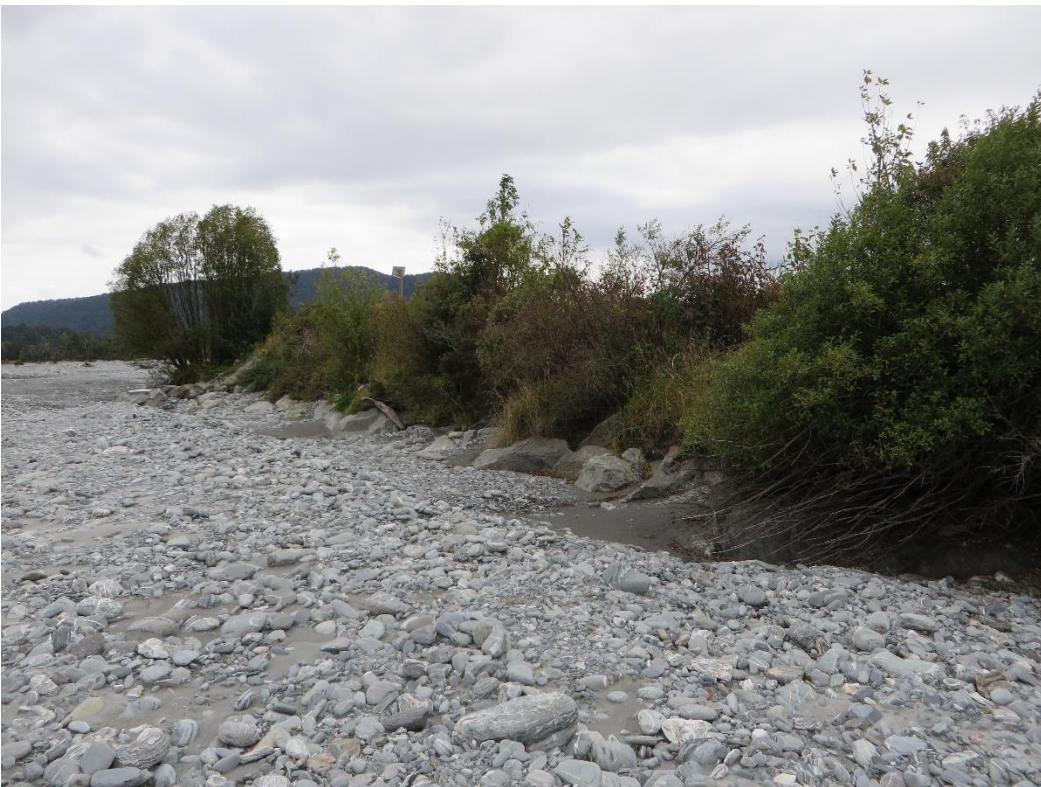
Figure 13: Partial submergence of toe of existing rock armour along embankment protecting oxidation ponds comprising Franz Josef Village WWTP
