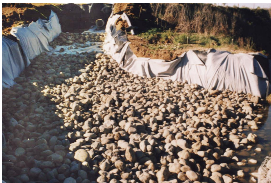
Figure 24: Example Rock Diffuser Discharge System under Construction (River at Right)
