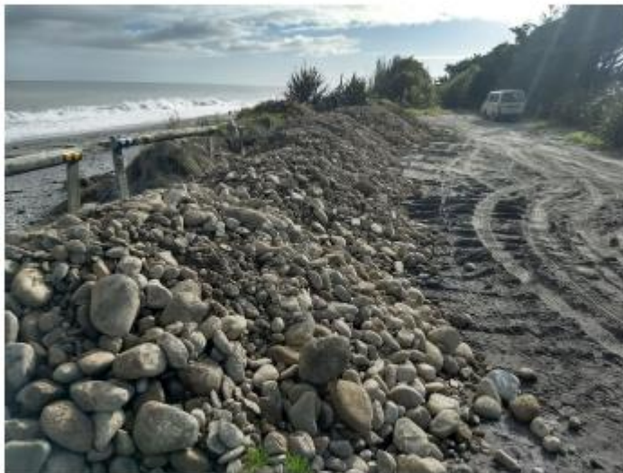
The erosion bund restricted access for parking already and may have to be increased in size in the near future
