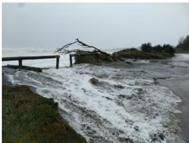
Coastal Inundation at the South Spit car park
