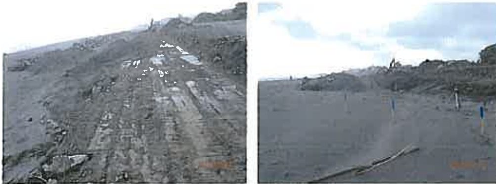
Hokitika Beach Protection – Initial Earthworks
