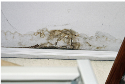
Leaks and cracking in the archive storage facilities.
