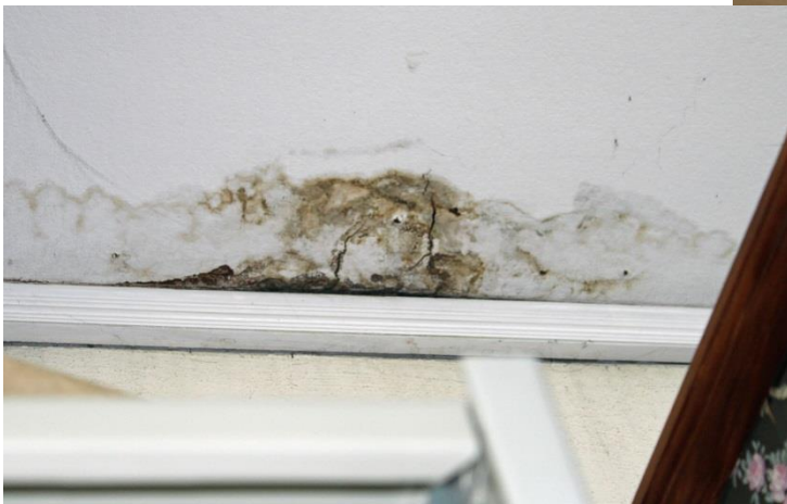
Roof leaks
