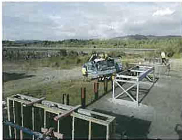
West Coast Wilderness Trail – Kapitea Spillway Bridge Construction
