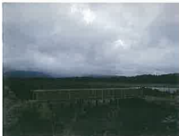
West Coast Wilderness Trail – Kapitea Spillway Bridge Completed
