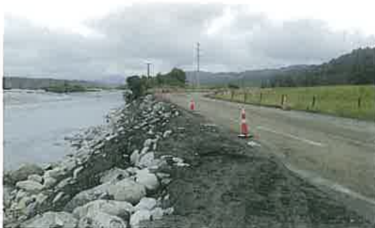
Washout Repairs – South Bank Arahura Road
