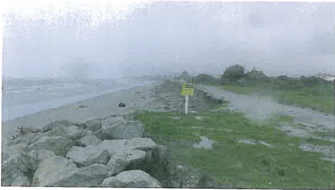
Figure 4: Eroding shore north of the short rip-rap seawall some 200 m north of the Tambo. 3 June 2013.
