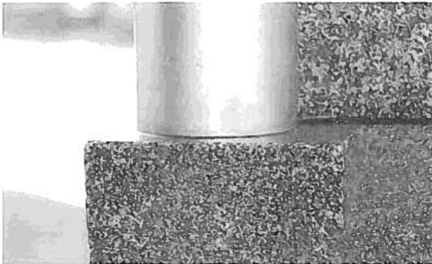
Algal growth on granite and rust around base of steel.
