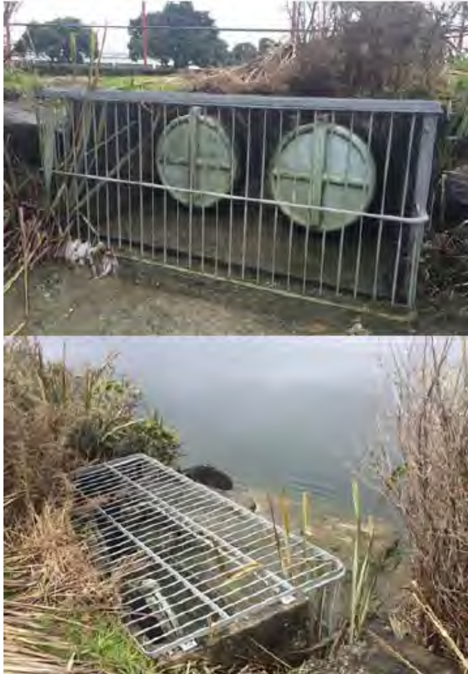
Figure 4-10 : Tancred St pump station discharge outlets to Hokitika River
