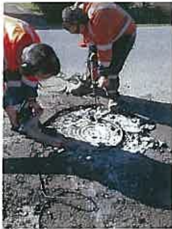
Wastewater Manhole Repairs Kaniere Road
