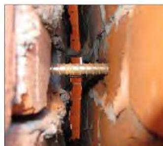
(c) Mechanical tie spanning cavity
