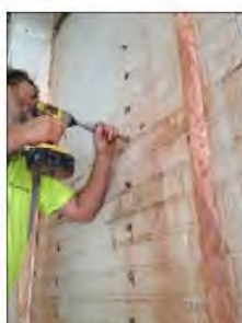
(b) Installing mechanical ties
