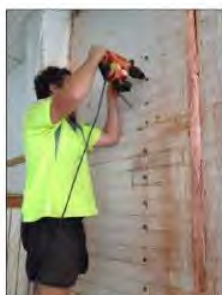
(a) Pre-drilling cavity tie holes
