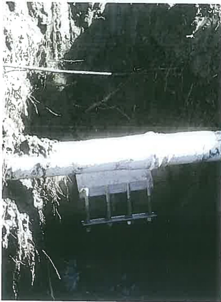
Hokitika Wastewater Pumping Main Split
