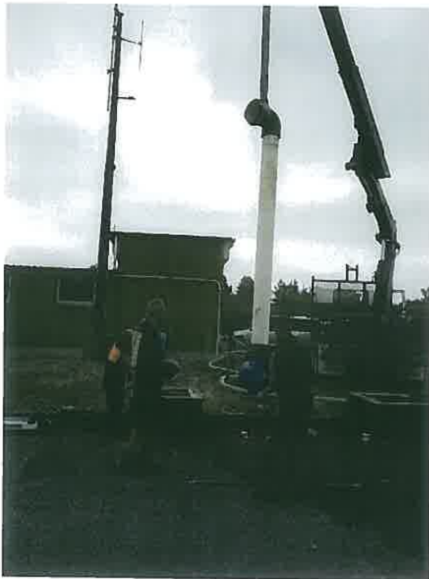
Brickfield reservoir – Foot Valve Repair
