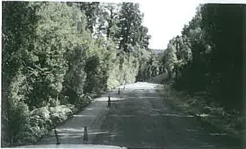
West Coast Wilderness Trail – Lake Kanieri Road Widening
