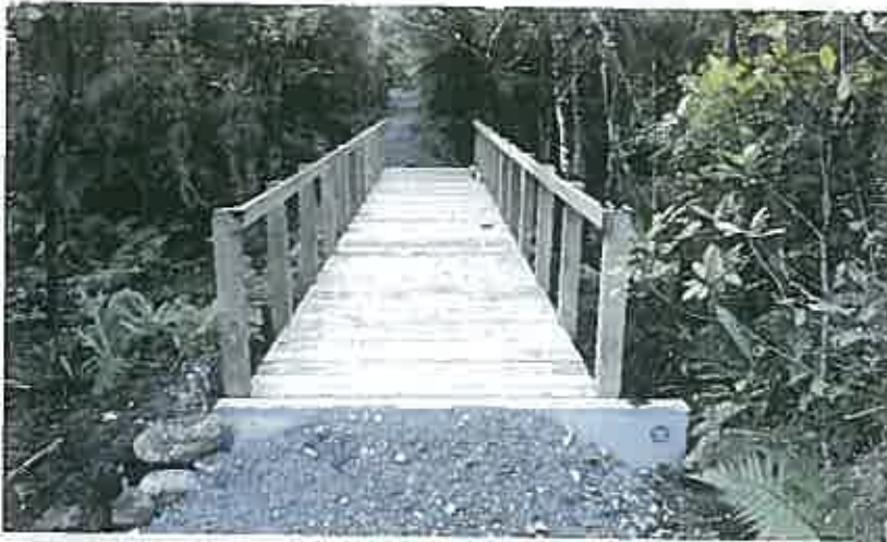
West Coast Wilderness Trail – Bridge Construction
