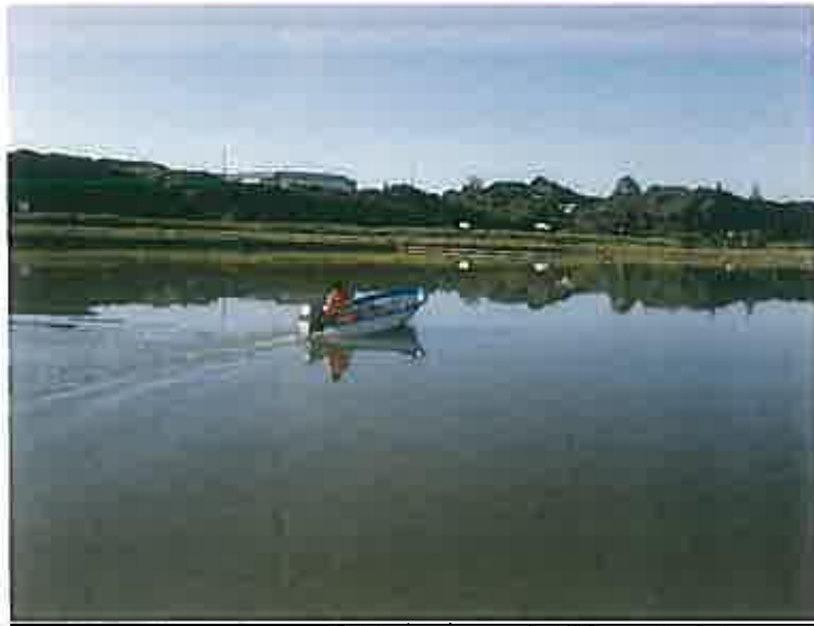
Hokitika Oxidation Ponds – Boat Aeration
