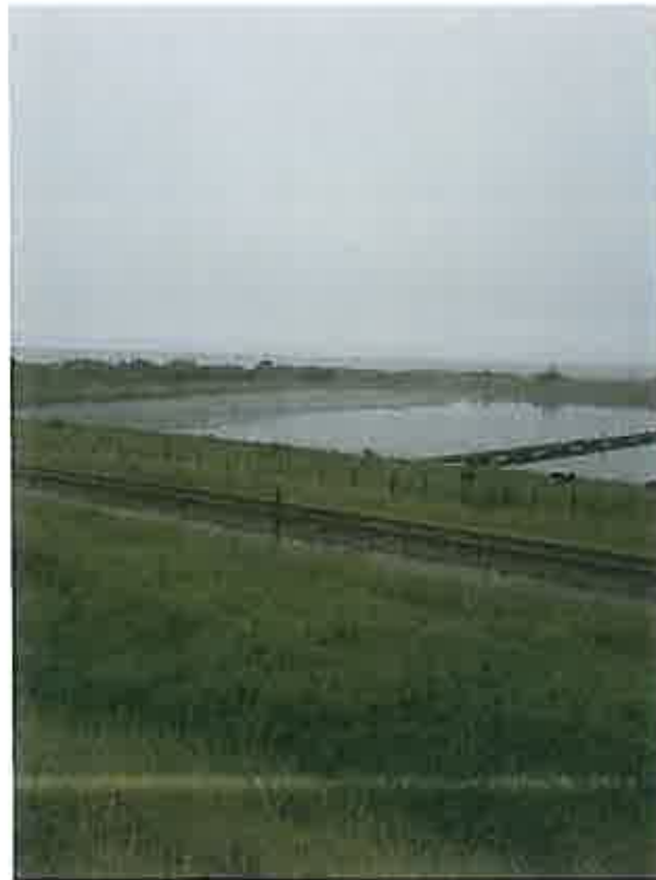
Hokitika Oxidation Ponds – Scum Build Up
