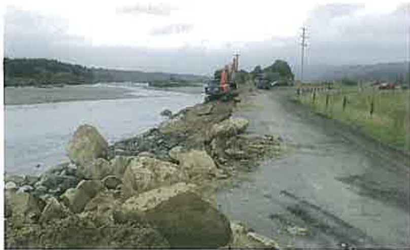
South Bank Arahura Road – Washout Repairs
