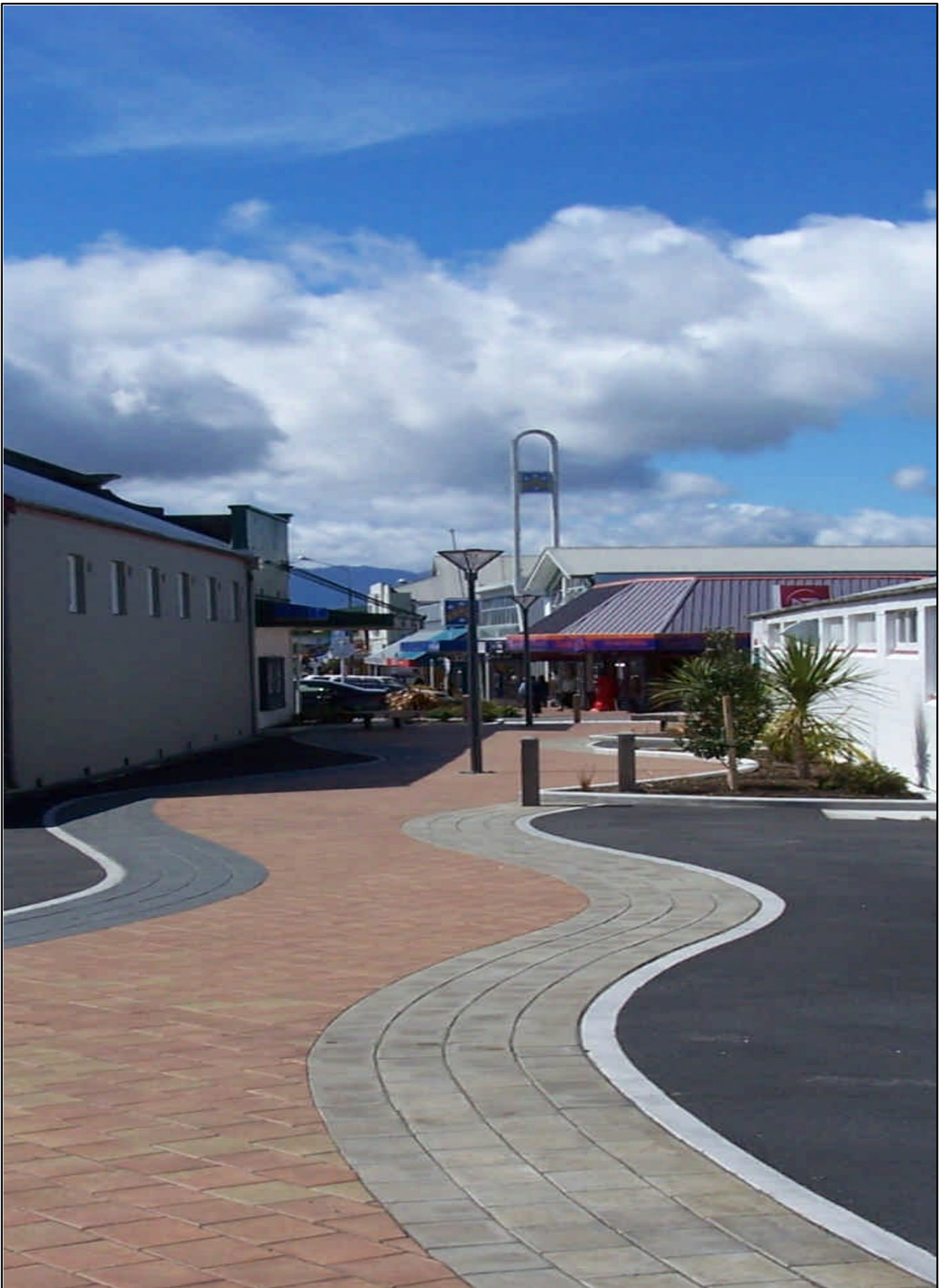
Stage One of Hokitika Concept Plan: Development of Weld Lane – Access from Township to Beachfront
