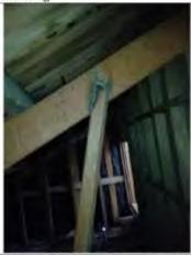
Diagonal web member re-welded to top chord following bending
