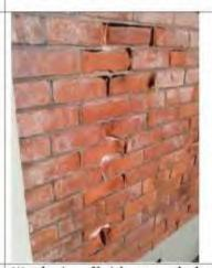
Weathering of bricks on north elevation
