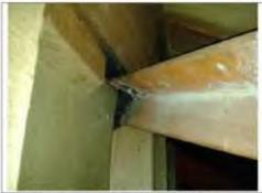
Angle brace cut and nailed to timber framing
