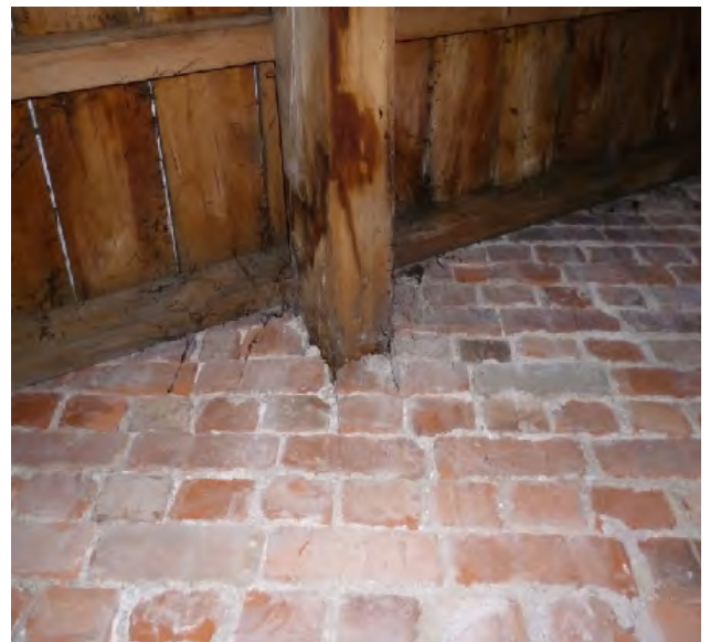
Photo 4 – Typical connection between purlin and gable wall
