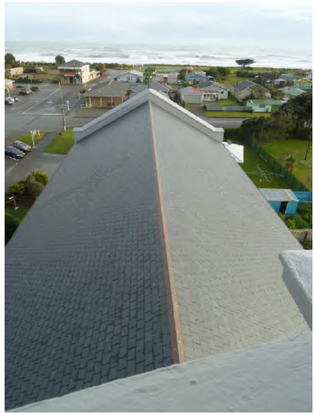
Photo 2 – Roof looking West
