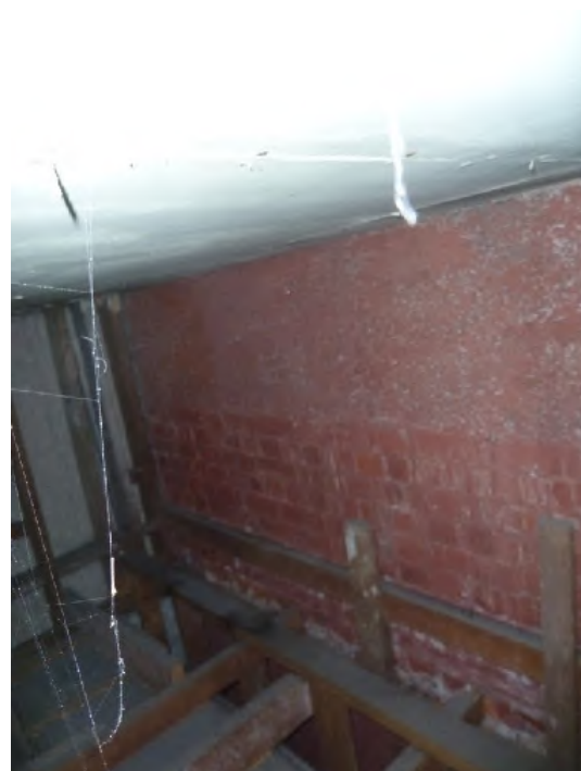
Photo 9 – Internal masonry wall sat on columns in photo 8
