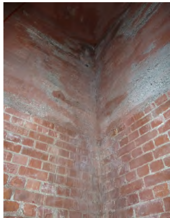
Photo 7 – Reinforced concrete tower sat on unreinforced masonry wall at mezzanine floor level
