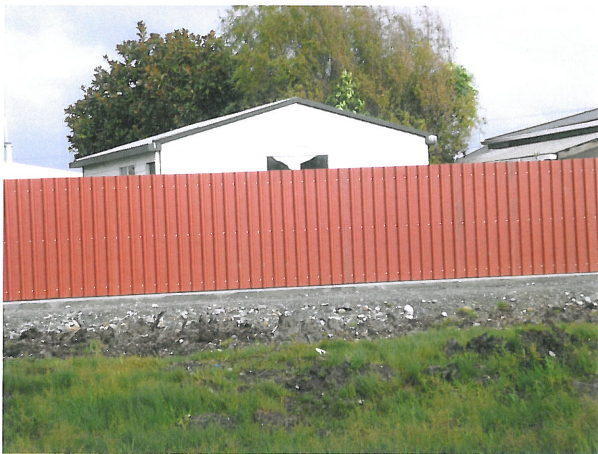
Part of completed fence
