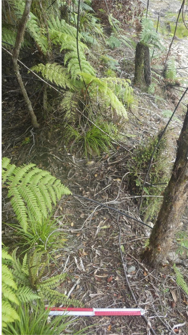
Figure 10. The water race berm, looking south, waypoint 142.
