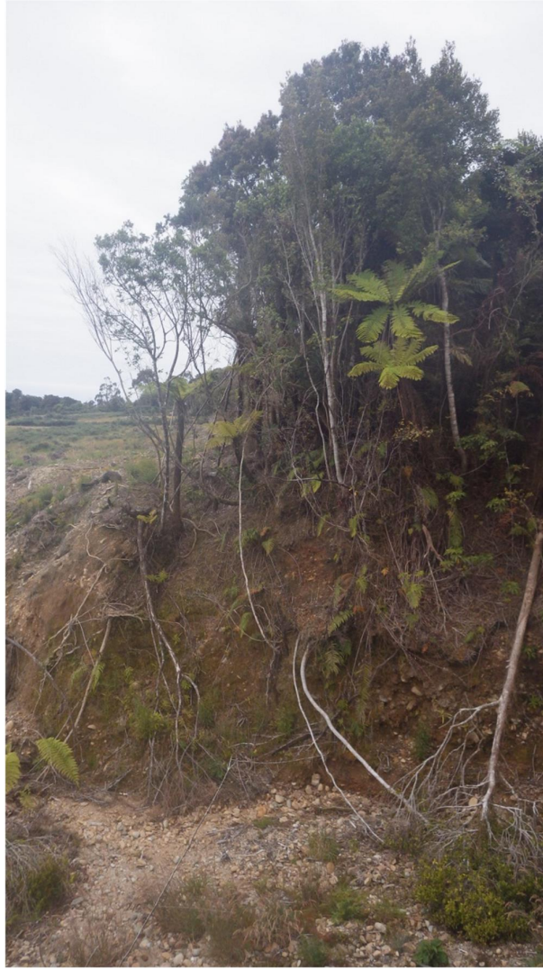
Figure 11. Looking northwest across Thistle Creek to the sluice faces on the true right of the creek, waypoint 144.
