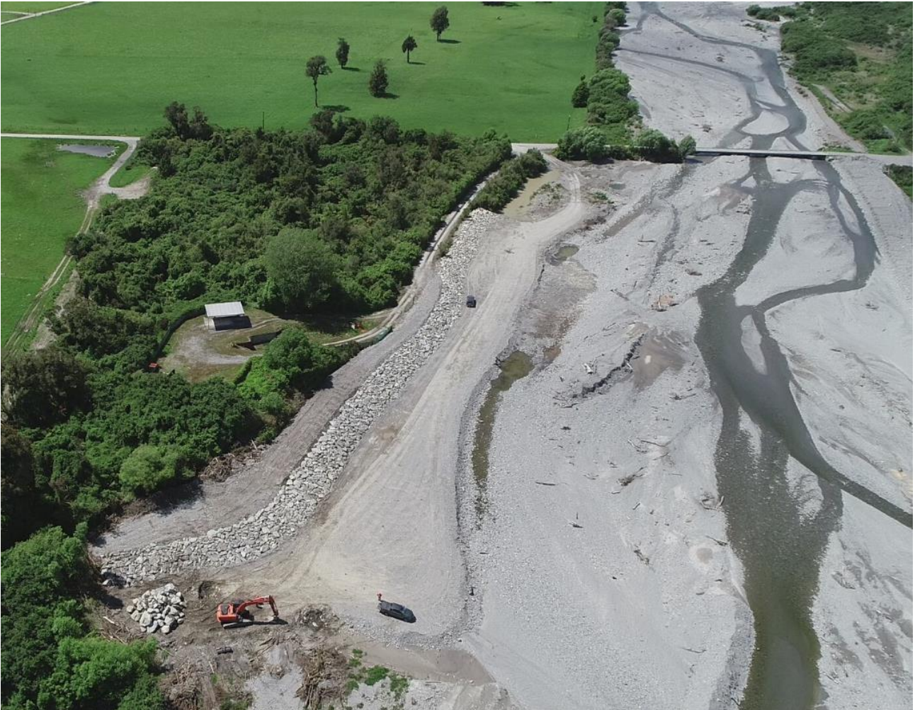
Figure 3-5: Rock Armouring Harihari Landfill.
