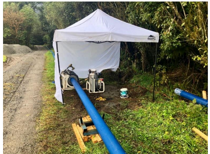
Fox Glacier Water Treatment Plant renewal work
