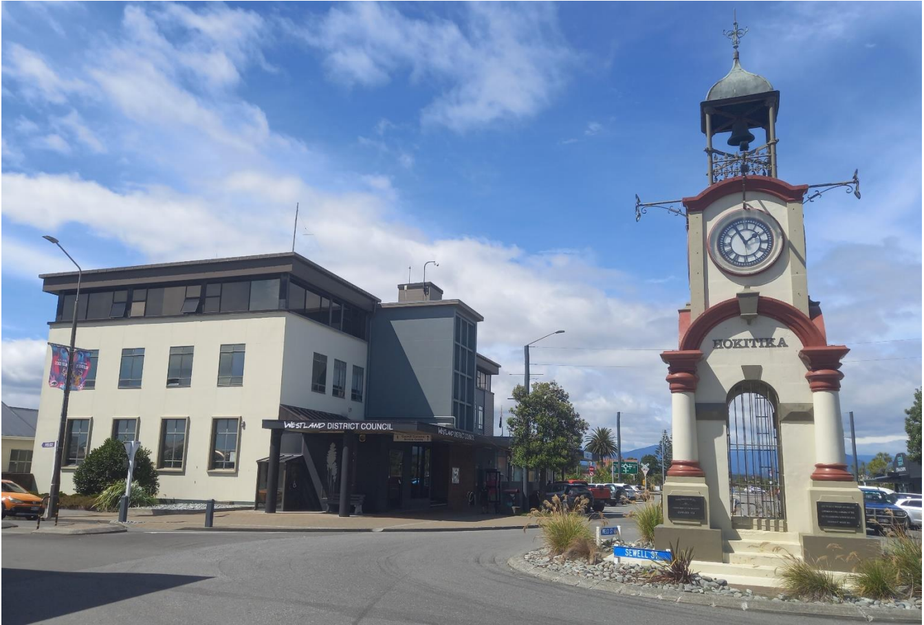
Westland District Council building
