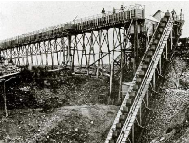
Impressive elevator plant on Donoghues
