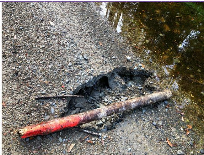
Figure 2: Typical Water Damage "Piping" to Trail
