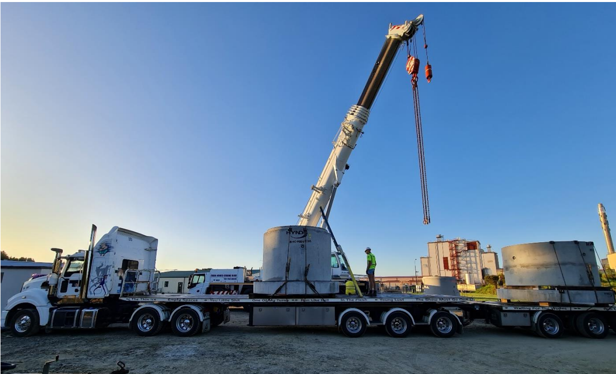
Figure: Town Belt East Stormwater Upgrade (February 2023).
