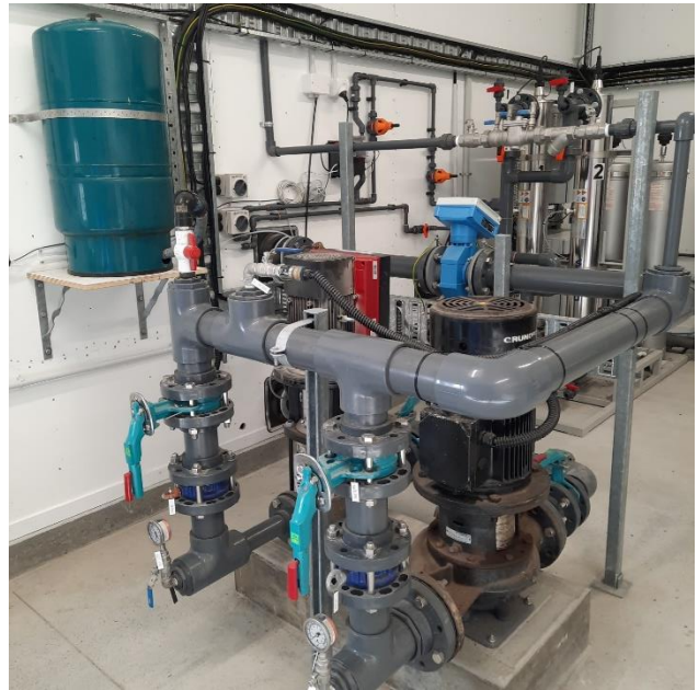
Figure 6-6: Reticulation Pumps.
