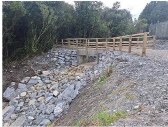
Major storms that occurred in May and June caused significant damage to various sections of the cycle trail. The Kaniere Tram box culvert got shifted from its base which caused a collapse of the headwall at either end making the trail impassable. As contractors were implementing the raising of river protection for regional council in a nearby area, they were utilised to undertake repairs and improvements. 100% MBIE funding was secured to undertake these works.
