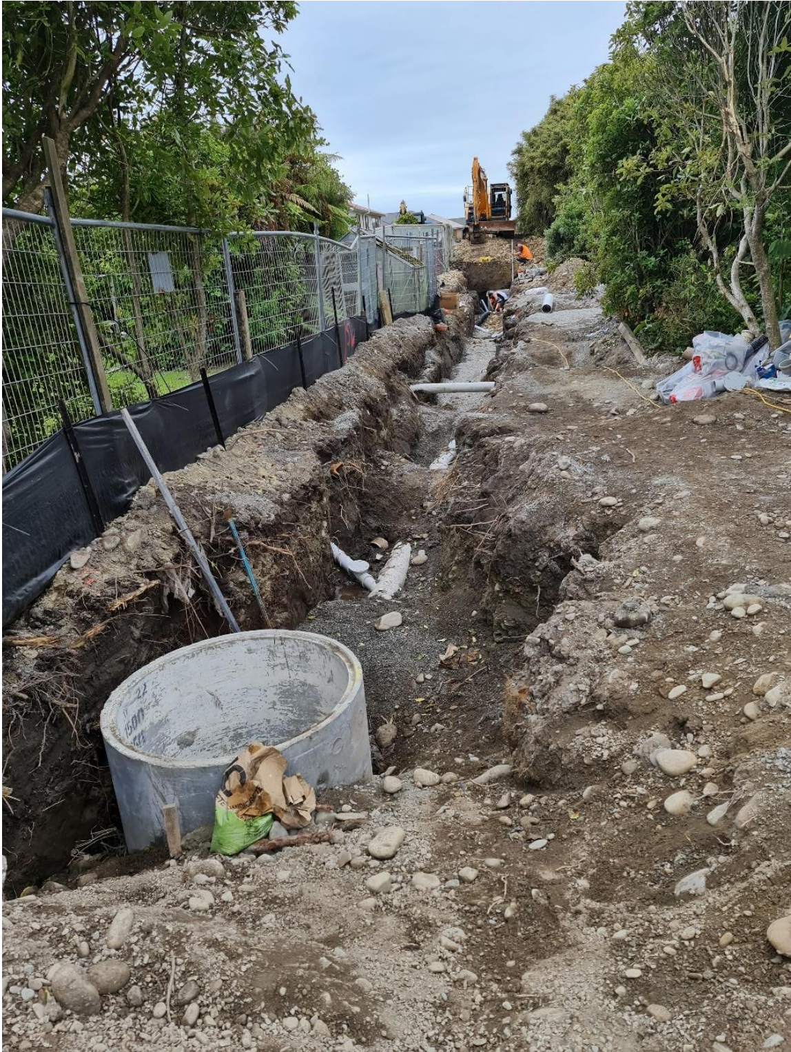
Figure: Hokitika Z-line Replacement (December 2022)
