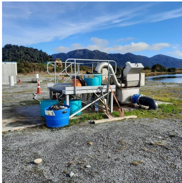
Figure 2-6: Septage Receiver.
