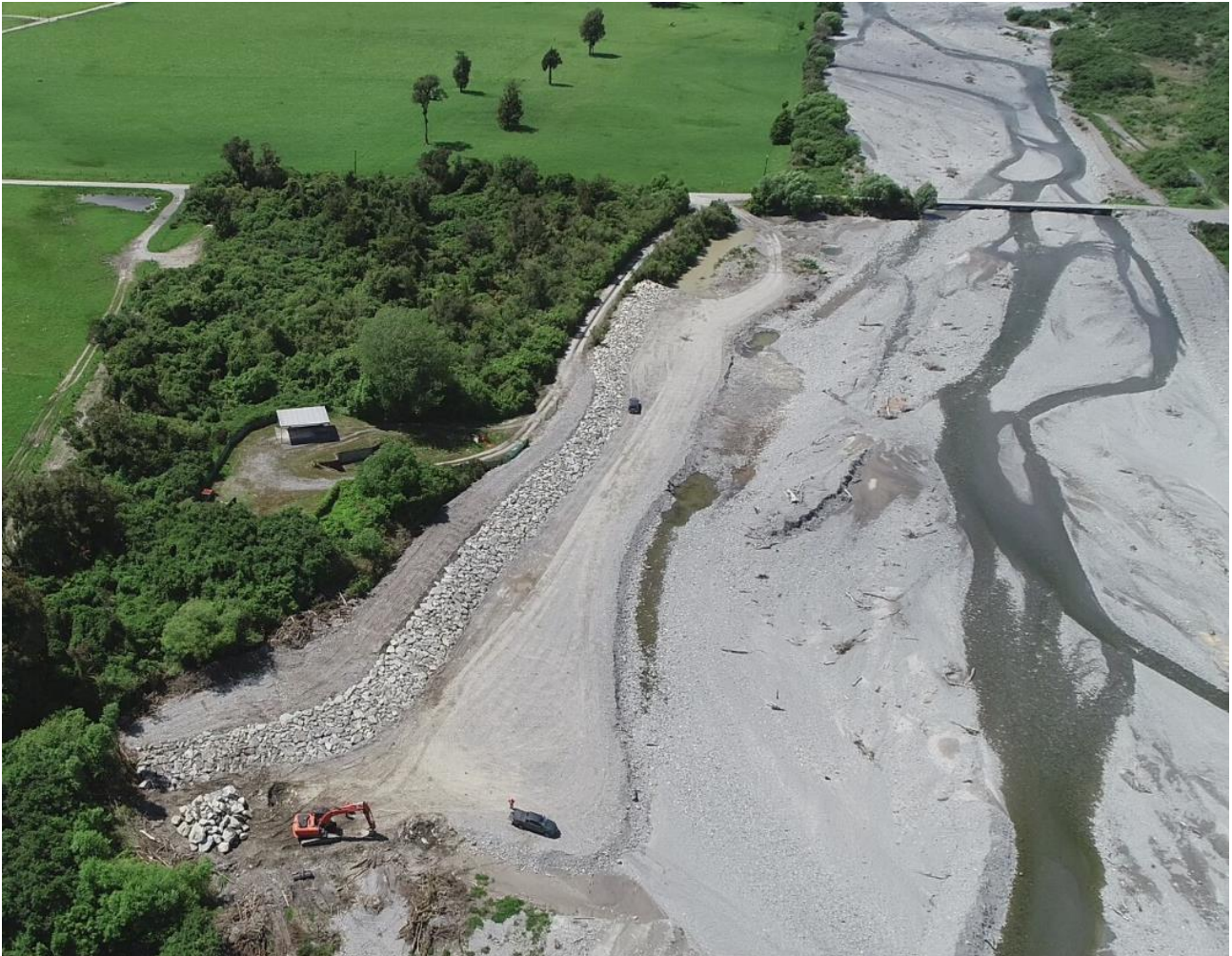
Figure 3-5: Rock Armouring Harihari Landfill.
