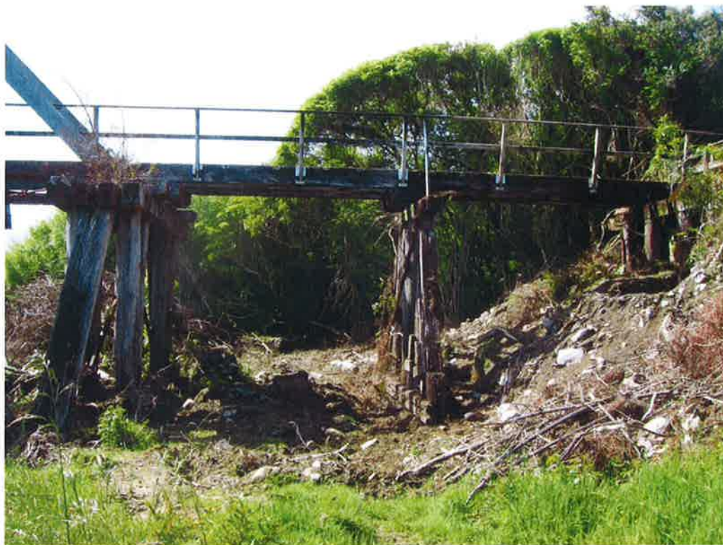
Figure 4-2 : Typical End Span (Spans 8 and 9 – Southern End)
