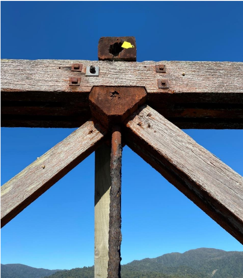
Saddle block with tunnel rot.
