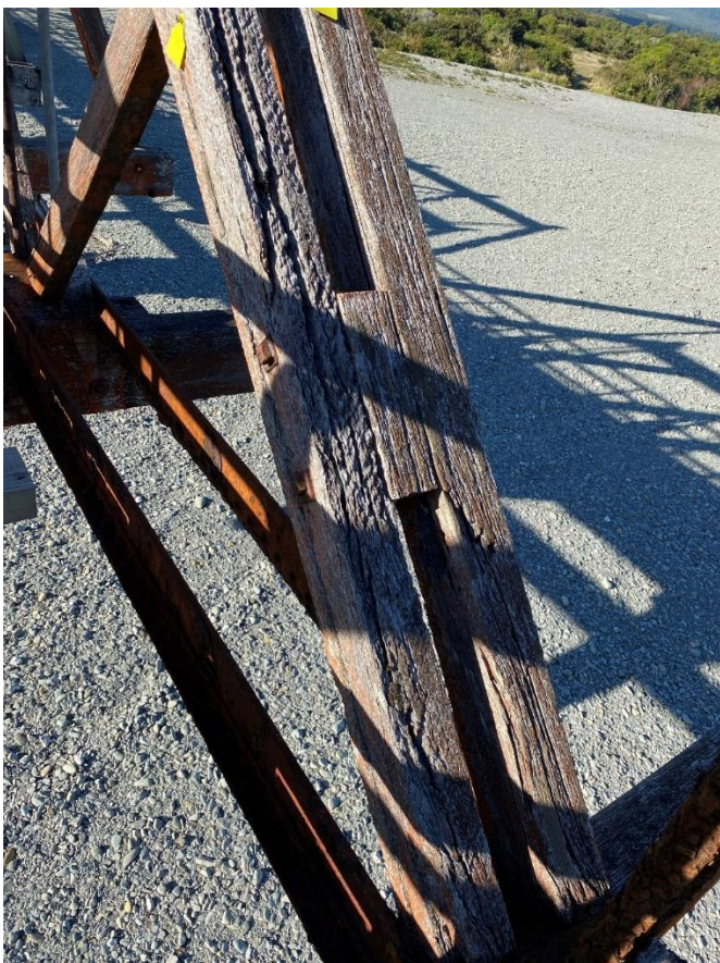
Surface loss on timber strut
