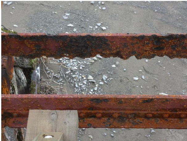
Moderate to Heavy Bottom Chord Corrosion.
