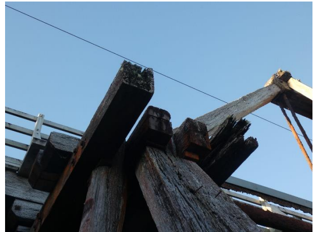
Typical Decay of Pier Cap Timbers
