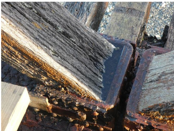
Typical Weathered Timber and Ponding Moisture.
