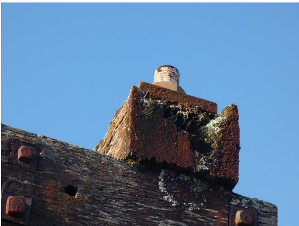
Typical Decay of Top Blocks.
