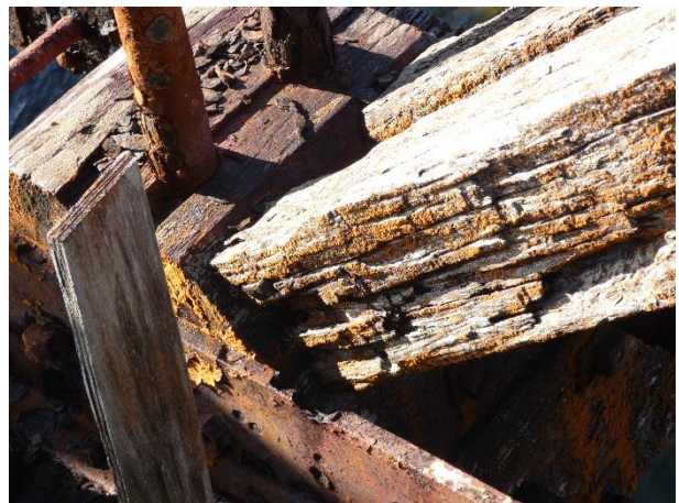
Typical Weathered Timber.
