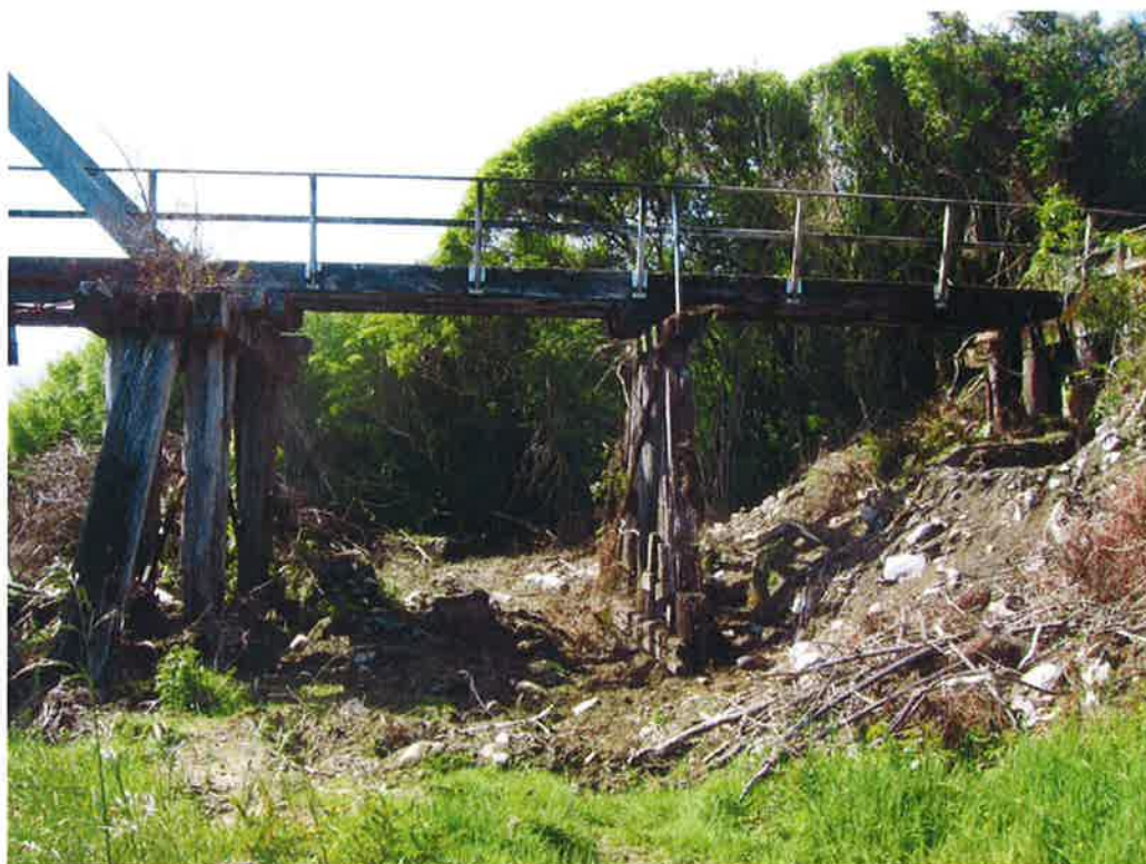
Figure 4-2 : Typical End Span (Spans 8 and 9 – Southern End)
