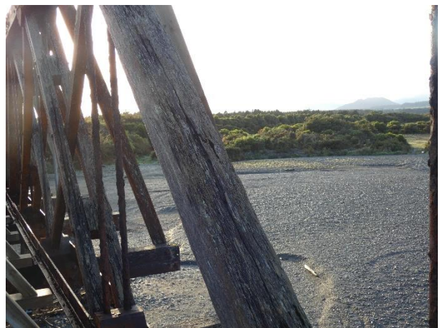
Typical Timber Splitting – King Strut Shown.
