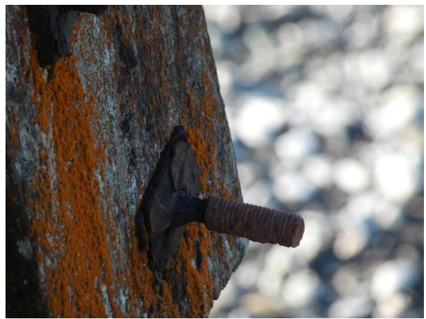
Corrosion and Loss of Fixing Components. Missing Nut and Necked Bolt Shown.
