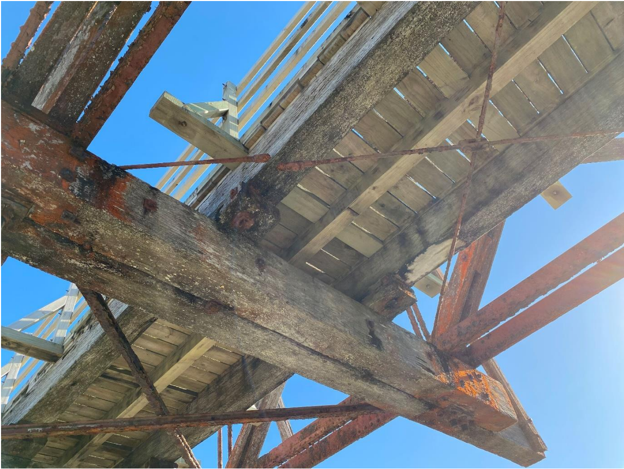
Cross bracing corroded away.
