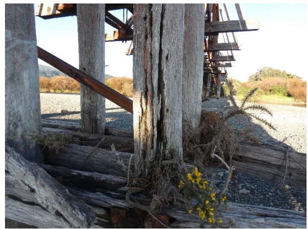
Typical Splitting and Decay of Pier Piles
