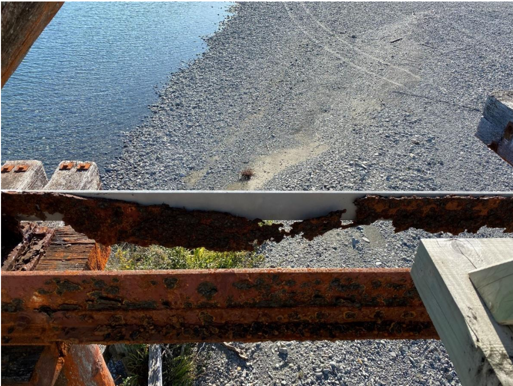
Bottom cord corroded. Previous repair visible.
