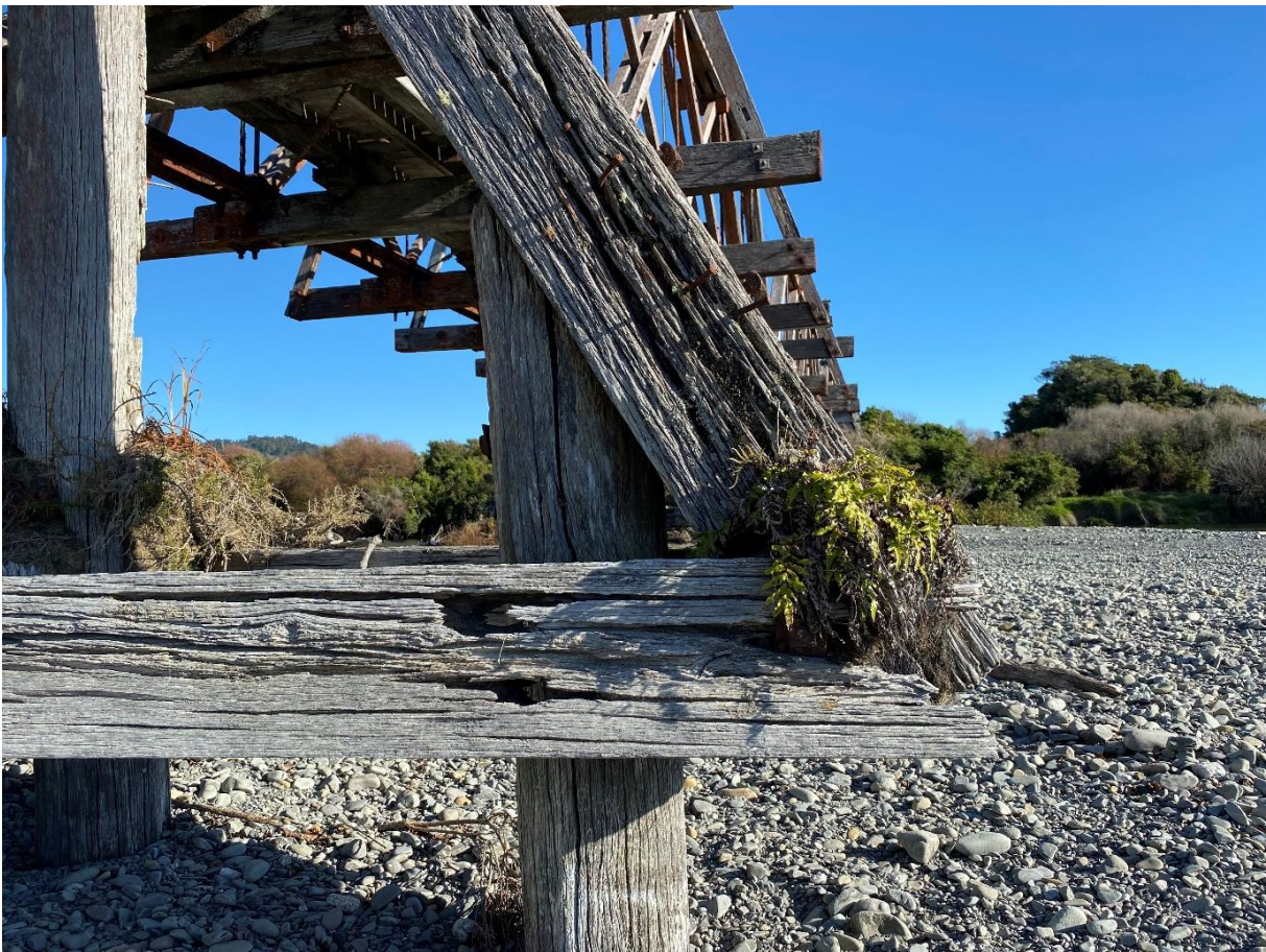
Timber loss and decay.
