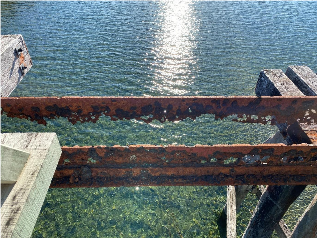
Bottom cord corroded. Needs replacing.
