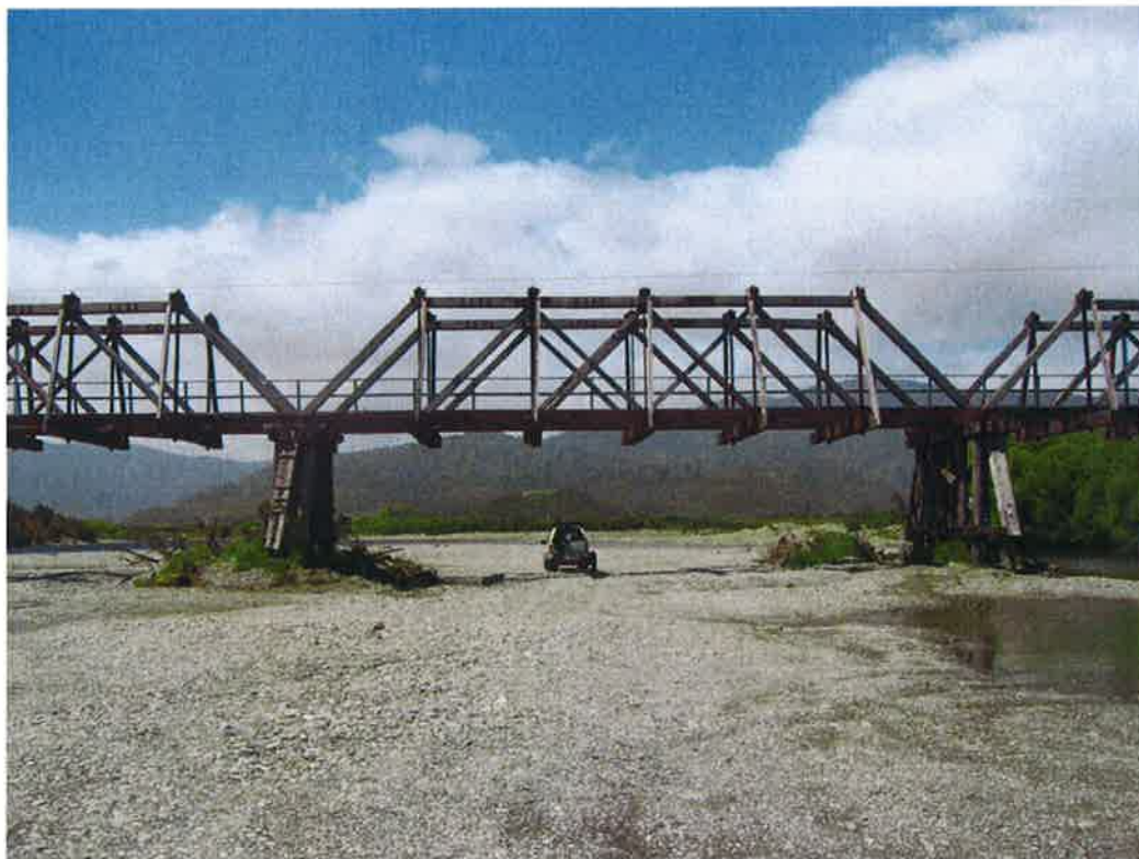
Figure 4-1 : Typical Howe Truss Span (Span 6 – Downstream)
