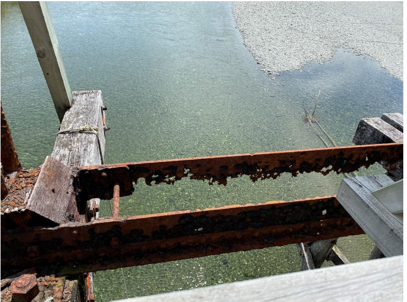
Bottom cord corroded, needs replacing
