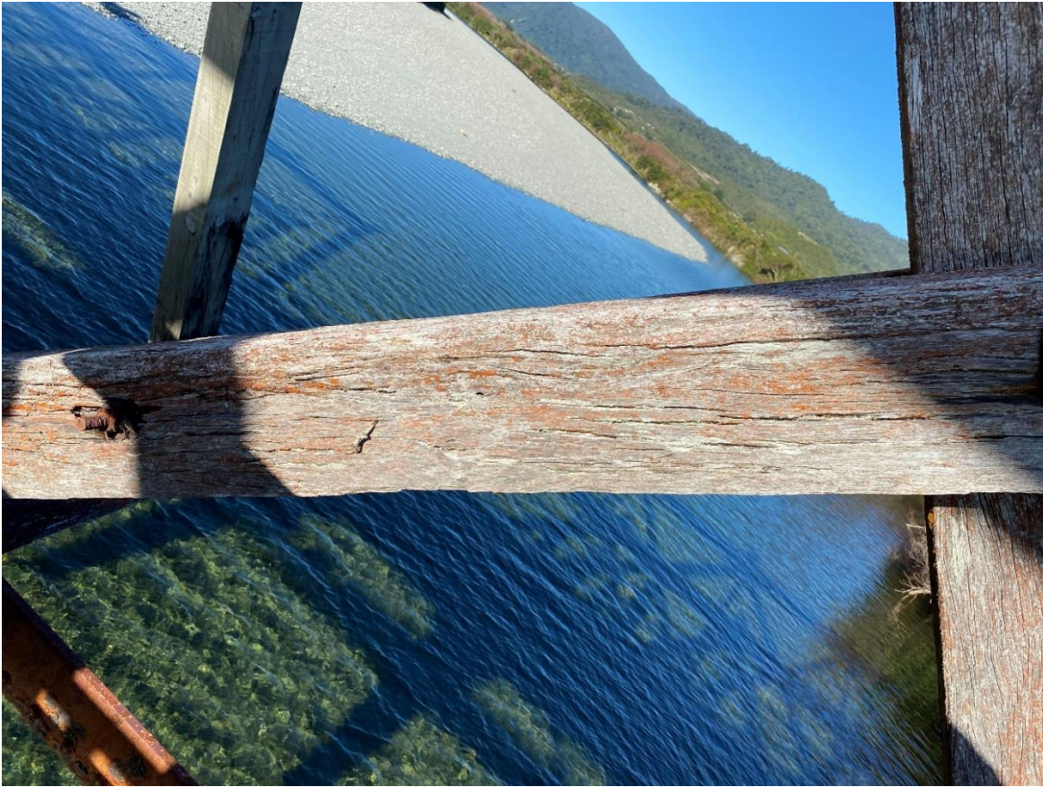
Centre strut timber decay.
