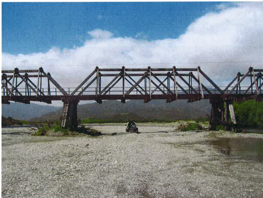
Figure 4-1 : Typical Howe Truss Span (Span 6 – Downstream)
