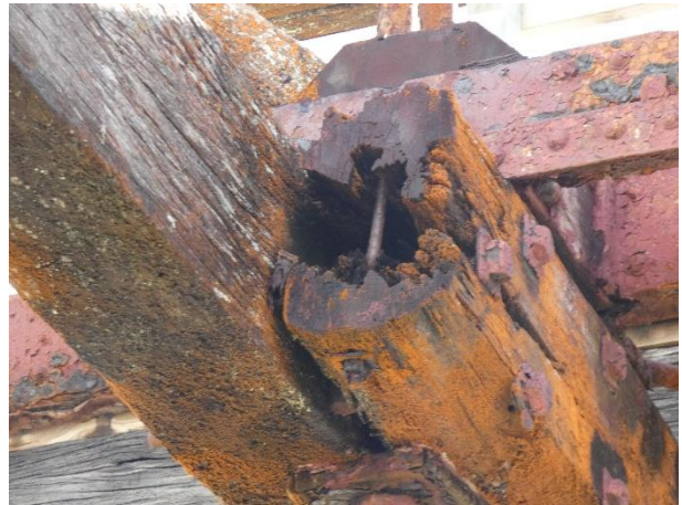
Timber Decay – Heavy to Critical Decay Shown.
