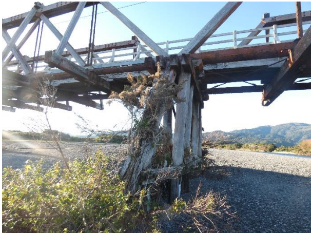
Vegetation Growth From Timber Decay Pockets
