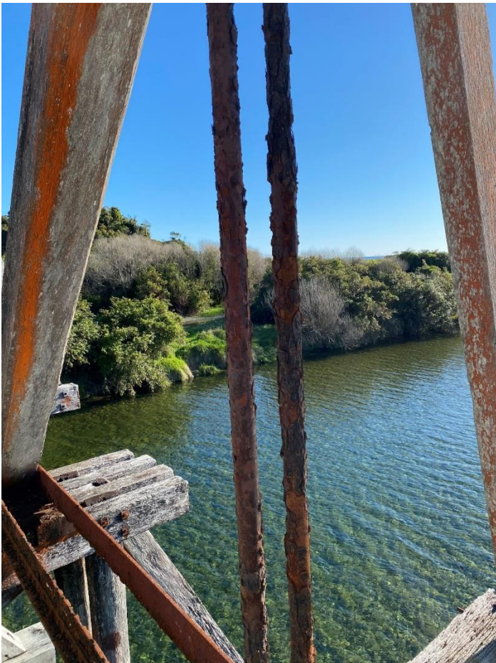
Tension rods corroded. Needs replacing
