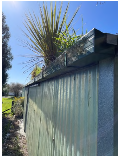
Gutter at South West Corner
