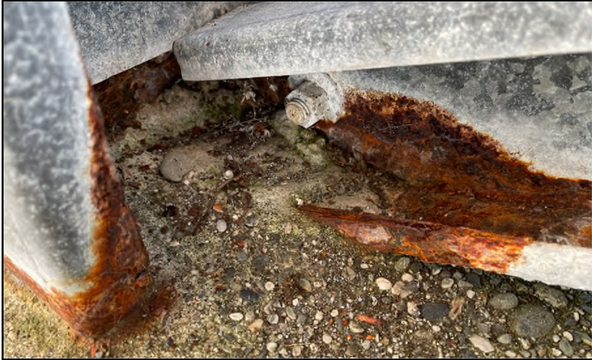
Photograph 13: Base of Portal Column and Brace at Grid Line 6
