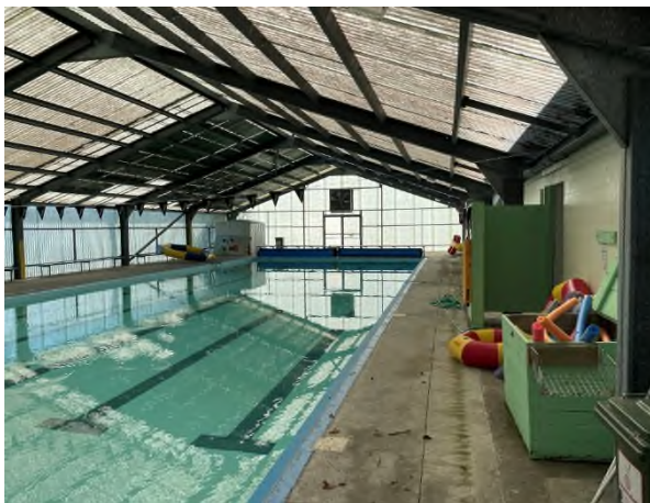
View to North
