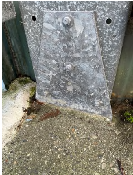
Portal Column Connection Grid Line 1
