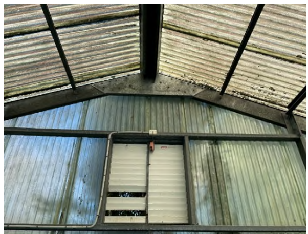
Apex Connection Grid Line 1
