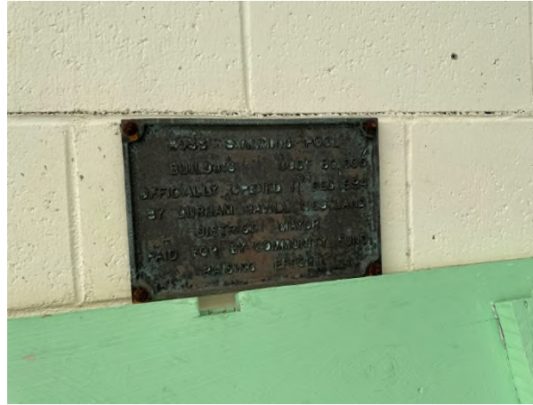
Horizontal Crack to Female Changing
