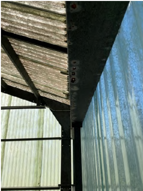
Holes in Girt Grid Line A
