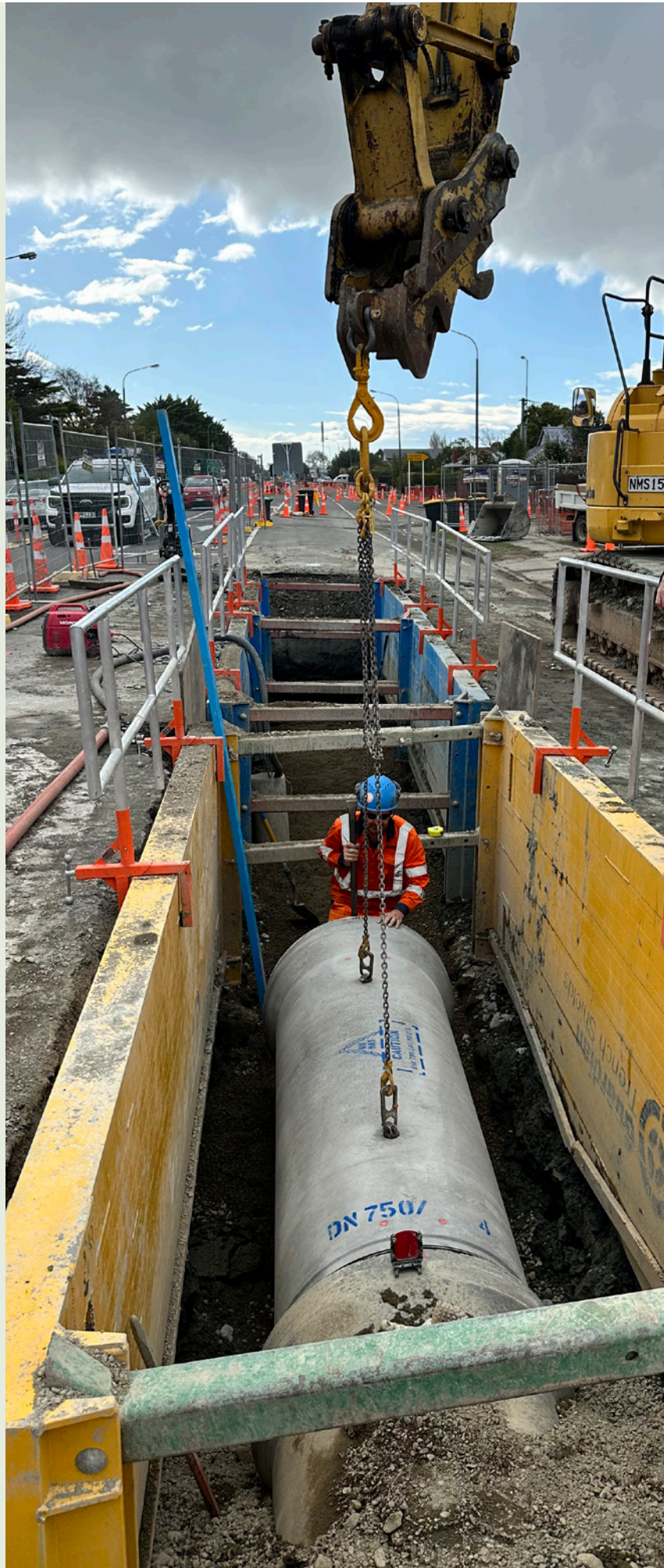
TD Crew working on the Halswell Road Drainage Job.
