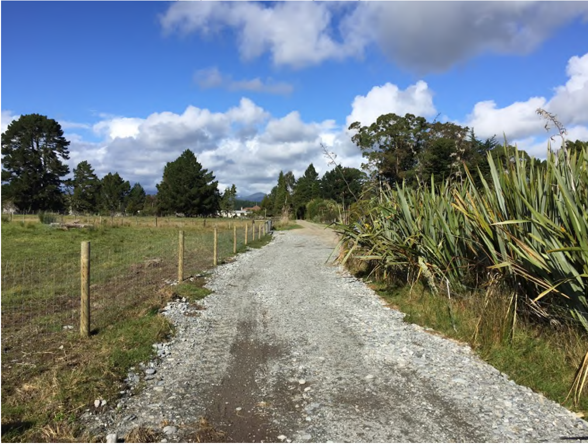
Hokitika-Kaniere Tramway Cycle Trail Fencing Realignment
