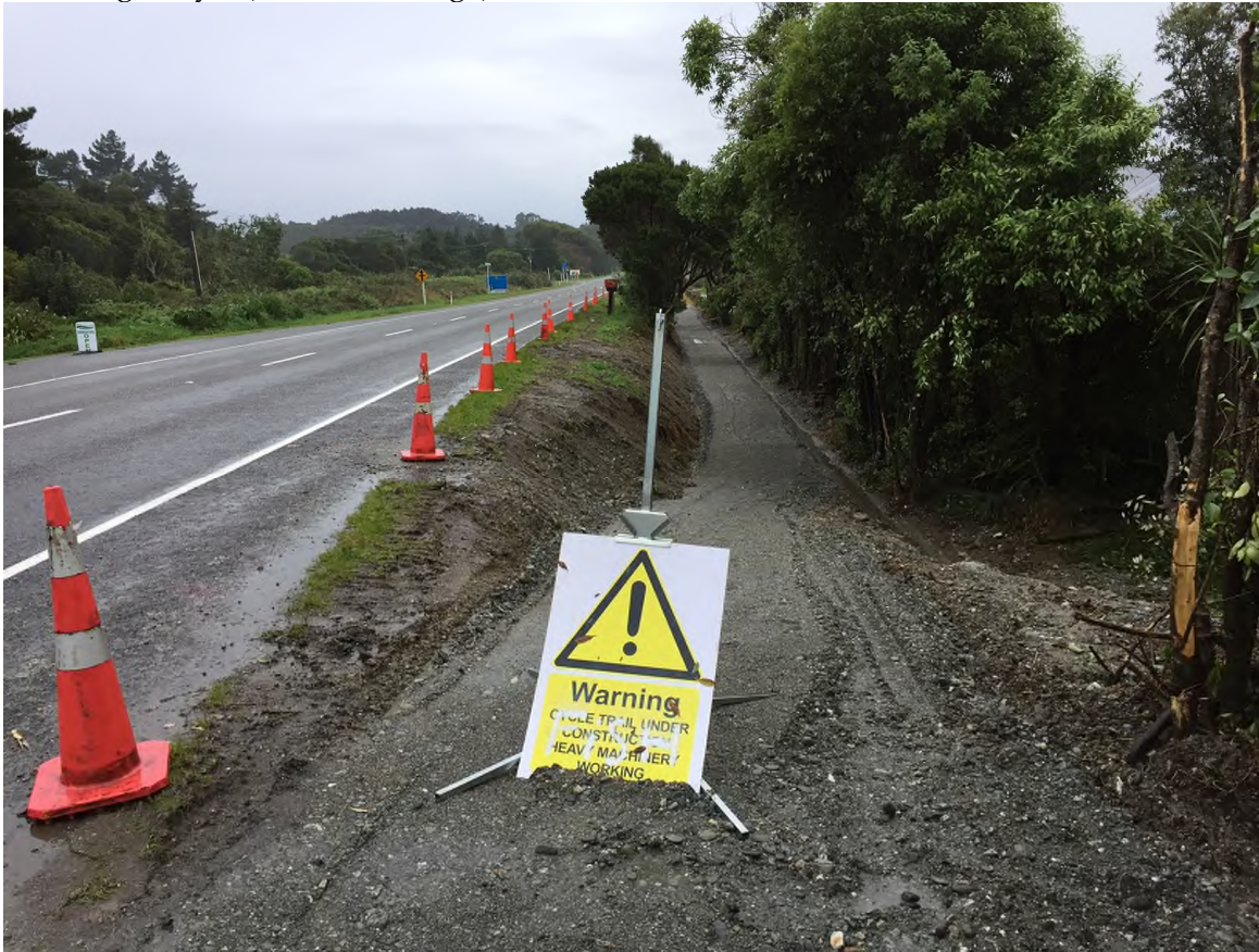
State Highway 6 (Hokitika Bridge)
