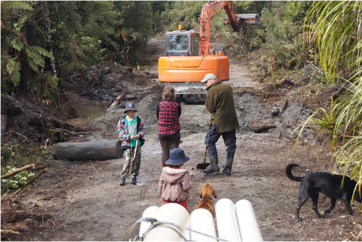
Photo 4 &5. Replacing rotting bridge with 1m diameter culverts and replacing old culverts along the logging road.
