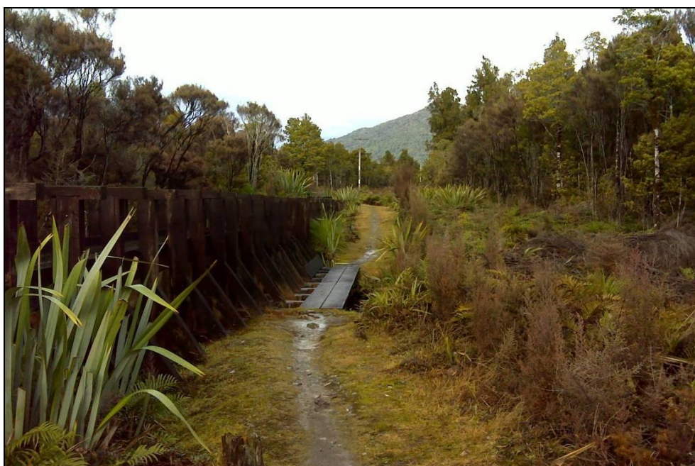
FIGURE 3.5.1 [EXISTING RACE WITH FLUME SECTION NEAR CHAINAGE 2600M]
