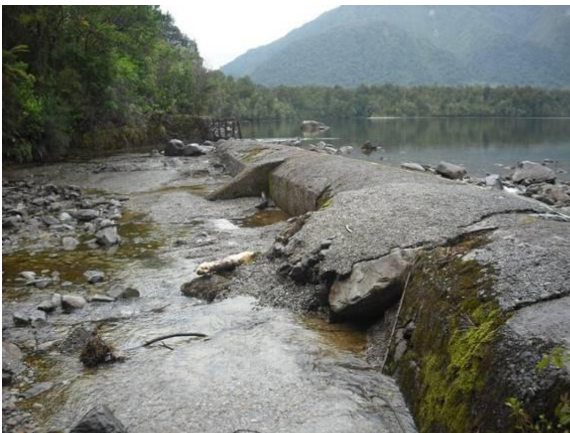
FIGURE 2.1.1 [LAKE KANIERE SPILL WEIR WITH STOP-LOGS]
