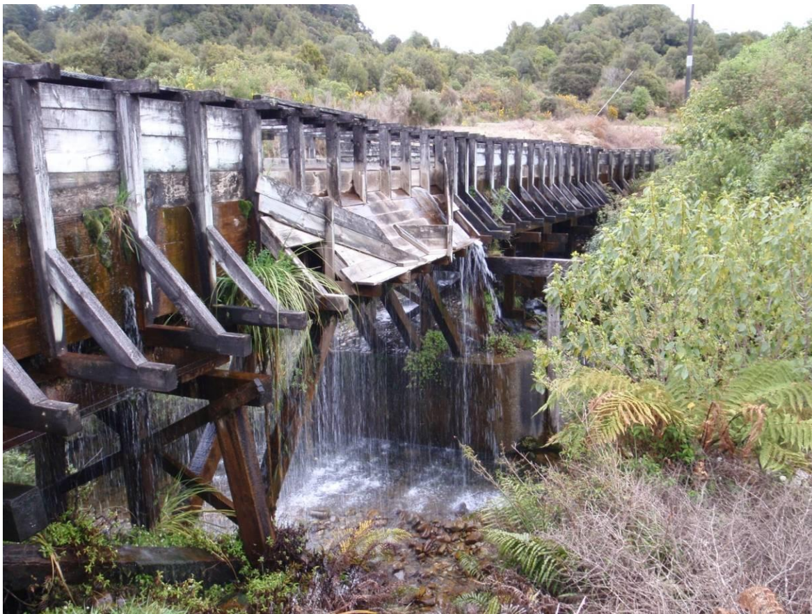
FIGURE 3.2.1 [COAL CREEK FLUME]
