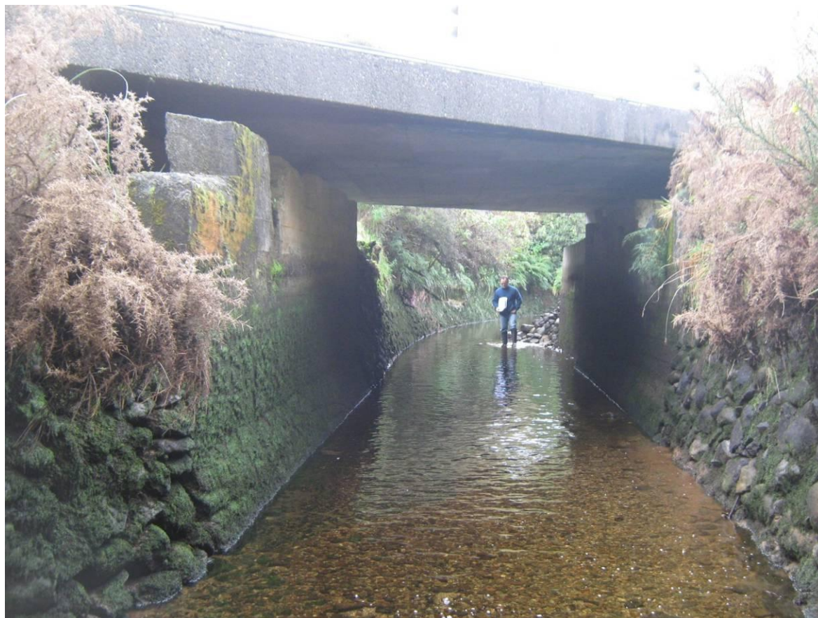
FIGURE 3.3.1 [MCKAYS WATER RACE AT KANIERE ROAD]
