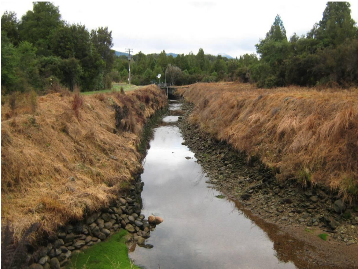
FIGURE 3.1.1 [MCKAYS INTAKE TO COAL CREEK FLUME]
